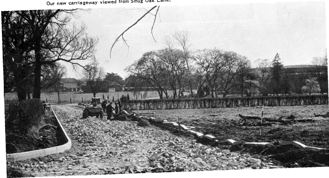
Our new carriageway viewed from Smug Oak Lane.
